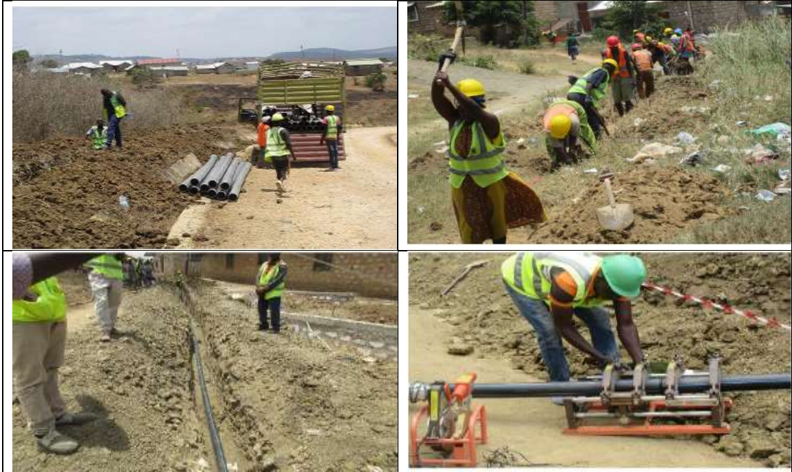
Figure 3-1: Construction and laying of pipeline
