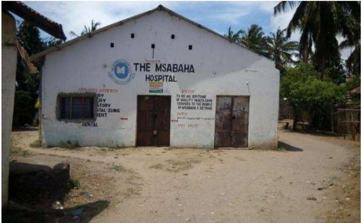
Figure 4-12: Health Infrastructure within Malindi Sub County
