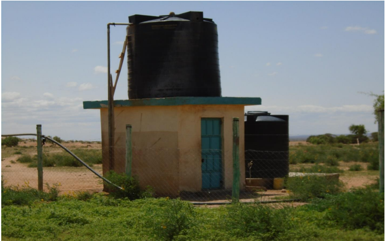
Figure 2-2 Raised plastic storage tank at the borehole at Ballah
