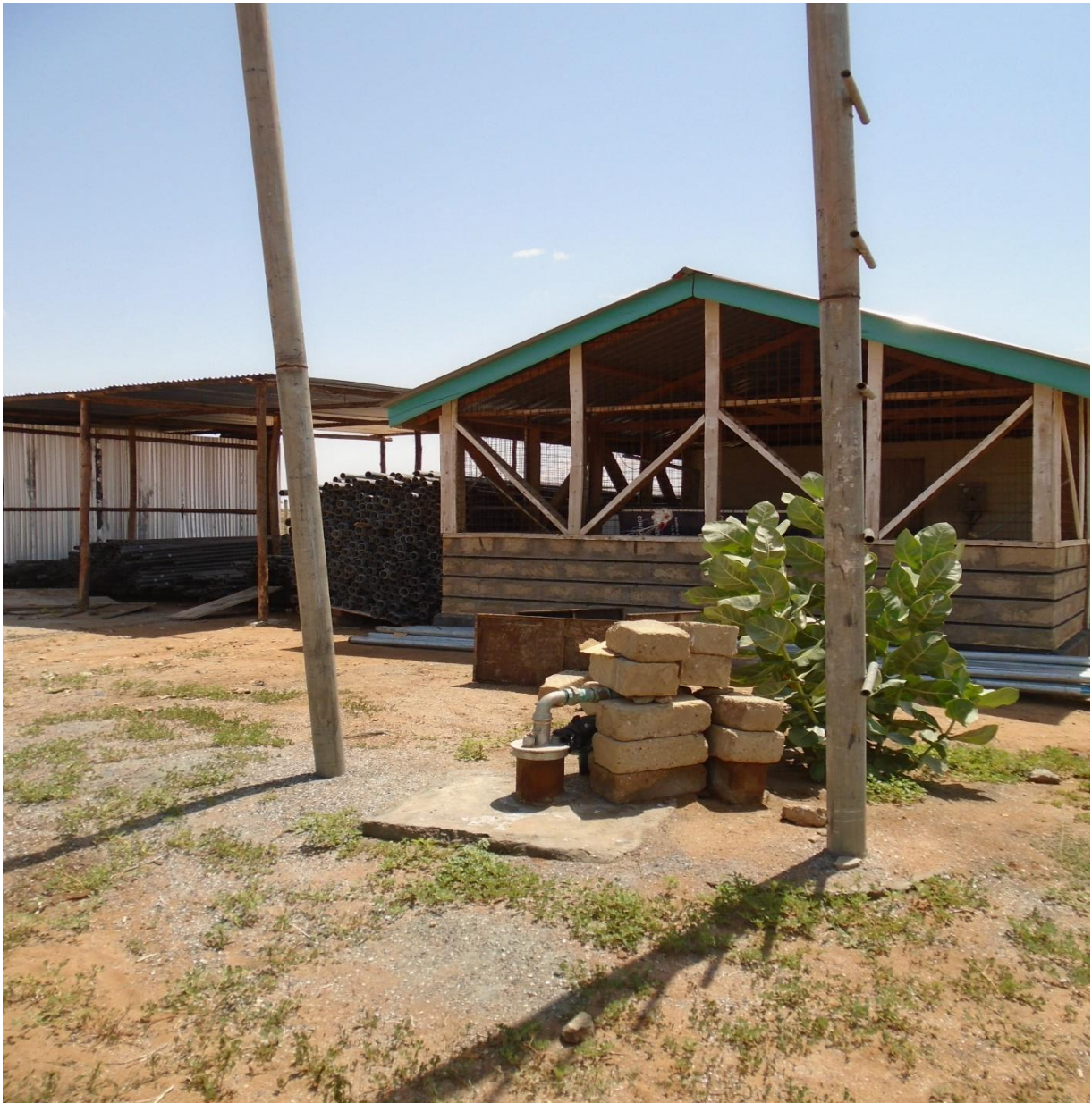
Figure 2-1 Borehole at Ballah
