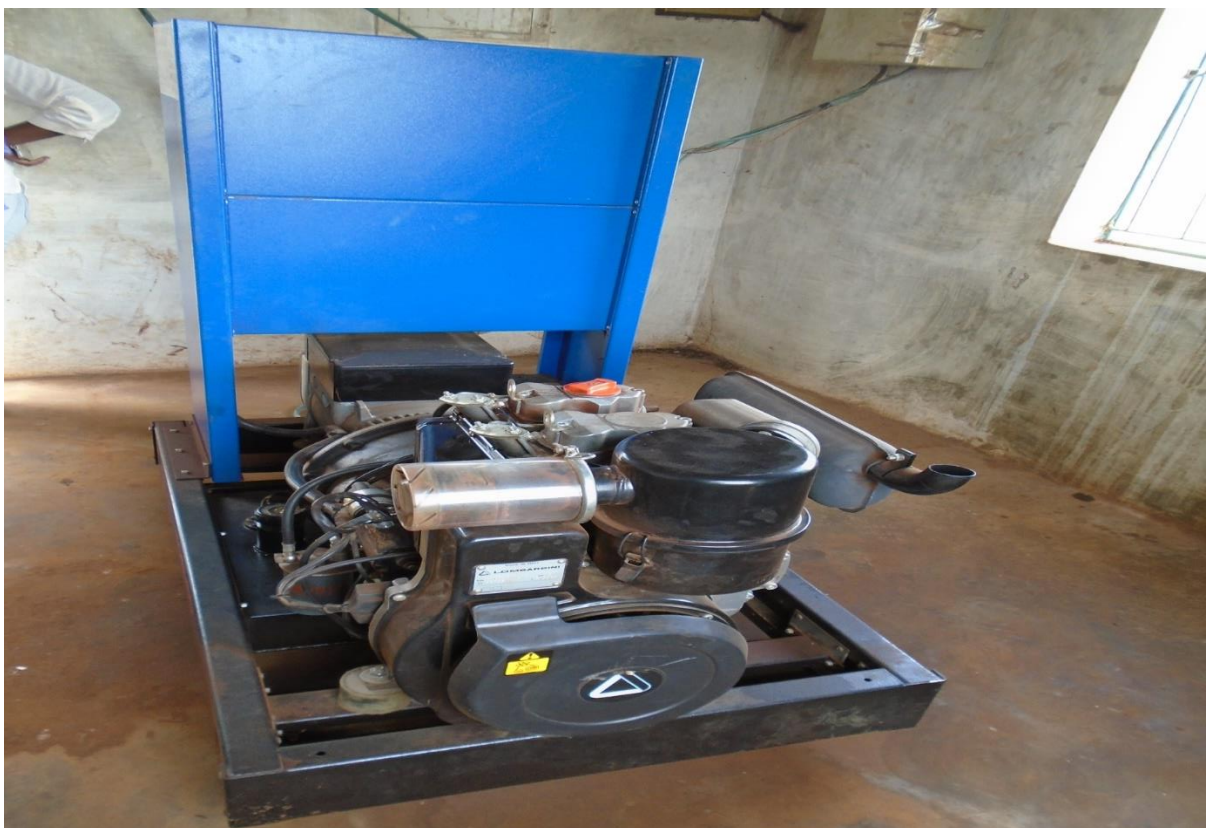
Figure 2-4 Standby Generator at Kachorandi 1 Borehole
