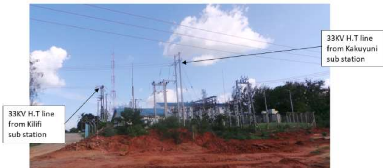
Figure 2-6: Baricho Water Works 33KV overhead H.T lines and substation
