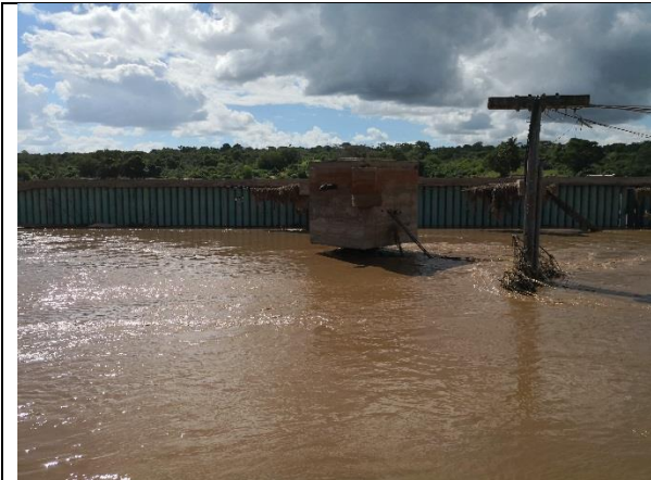
One of the damaged boreholes (Borehole no. 3) and the then protection surrounded by the flooding water
