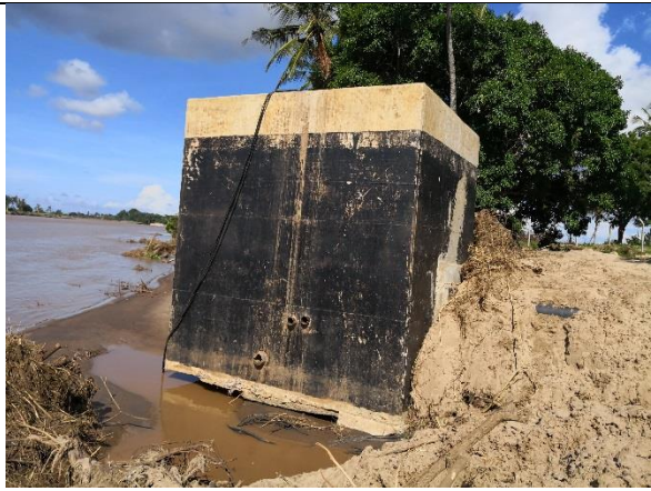
One of the recently constructed borehole (no.11) which was still under construction during the flooding
