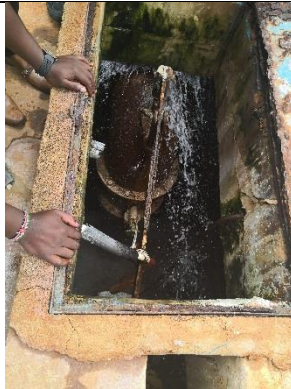
Damaged borehole electrical fittings
