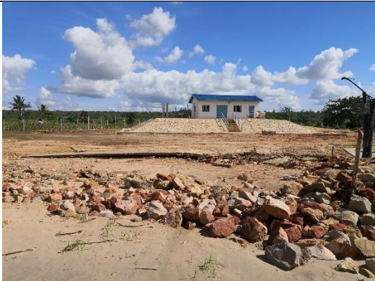
The new transformer house after flooding
