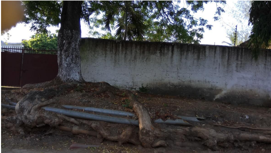
Figure 4-4: Relationship between some trees and existing infrastructure
