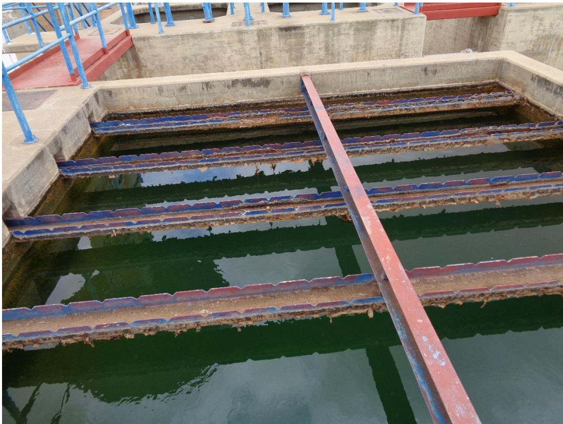
Figure 2-3: Clear Water Tank
