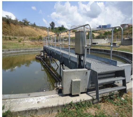
Providing Human Dignity - Rehabilitated sewerage systems
