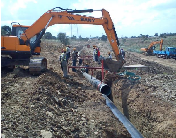
Sustainable development – Replacing a pipeline
