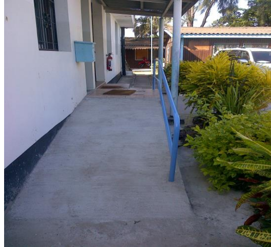
Caring for the marginalized - Ramps for the physically challenged
